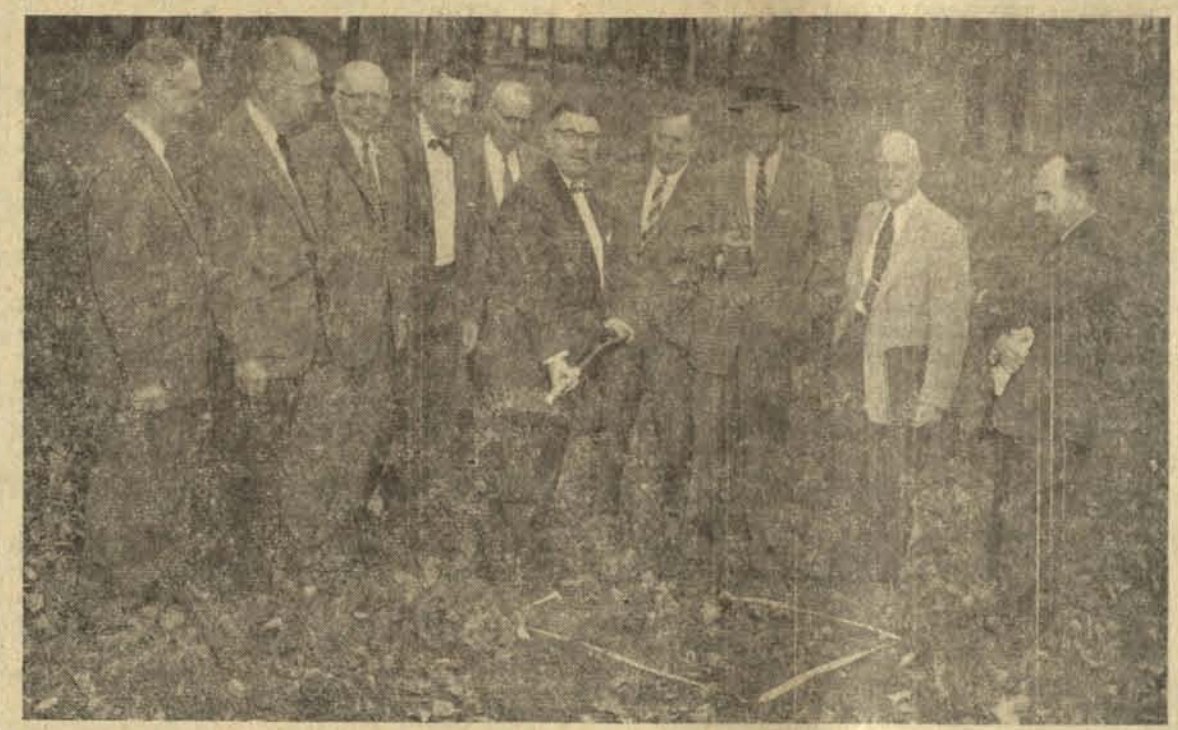
MERRITT CHROUCH, general manager of United Cooperatives, Inc. and the board of directors took part last month in ground breaking ceremony for a new office building at Alliance, Ohio, where United has been since 1942.
