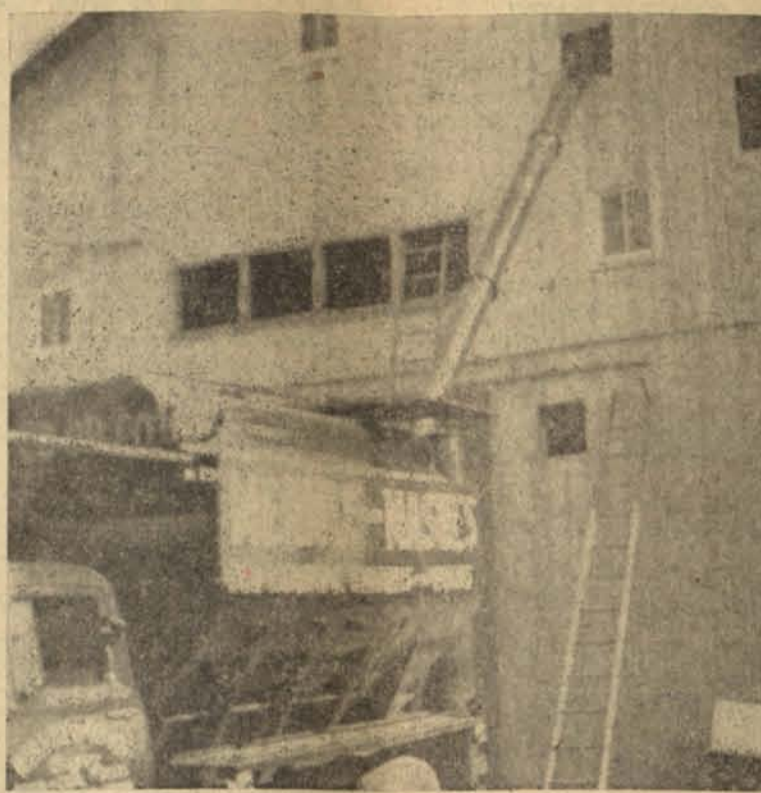
BULK FEED DELIVERY UNIT of the Holland Cooperative Company is shown making delivery of Farm Bureau HI-N-R-G Broiler Mash to the Leon Scholten farm near Holland. A 20 ft. auger raises feed for 4,000 caponettes to the bins. The seven ton capacity truck has three compartments to permit delivery of different feeds. Louis Van Huis, manager at Holland, says bulk delivery saves time and money for the farmer. He doesn't have to handle bags or even be there when the delivery is made. The cost of bags is eliminated.
