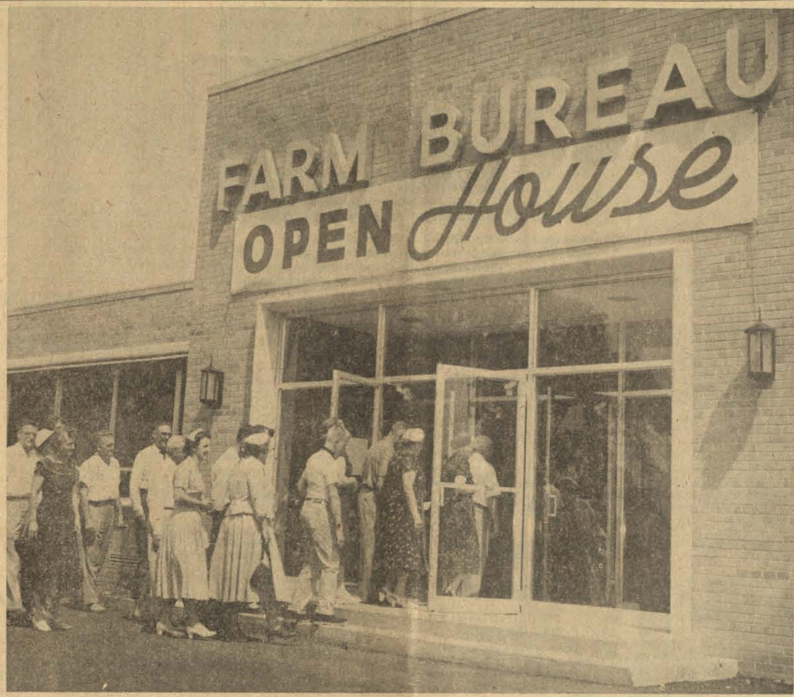
THIS IS THE WAY the front entrance of the Farm Bureau building looked August 10 as groups of Farm Bureau members came for the Open House. They registered at the lobby desk and proceeded on guided tours throughout the building. Afterward they had picnic lunch in the big tent pitched behind the office building, then participated in the dedicatory program in the afternoon.
