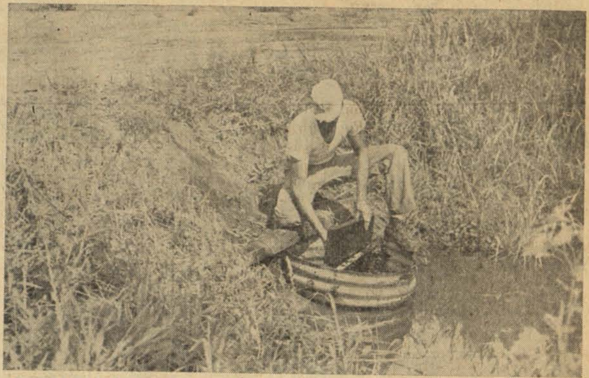
ROBERT HANSEN places a plank in the spillway to form a dam that controls the depth of water in the drainage ditch. By raising or lowering the plank dam, the water level can be raised or lowered in the fields adjacent to the ditches.
