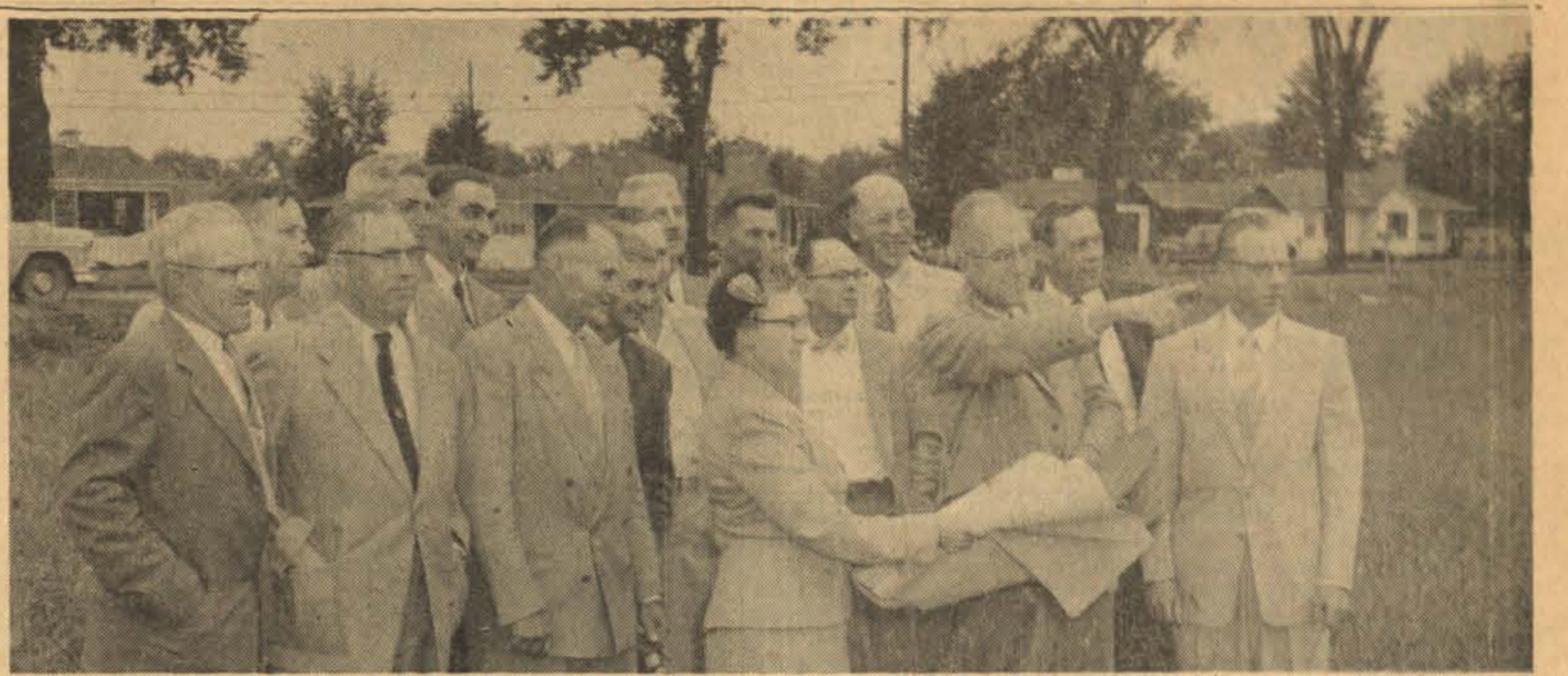
J. F. YAEGER, executive secretary of the Farm Bureau Insurance Companies, and directors are shown on the site of the new Farm Bureau office building at 3900 North Grand River Avenue (US-16) west of Lansing. Mr. Yaeger is explaining construction features of the building. In the background is US-16 and the residential area the offices will face. The building will be set back considerably from the highway. The area in front and right and left of the building will be landscaped to add to the appearance of the offices and to screen the rear parking areas from the highway.
