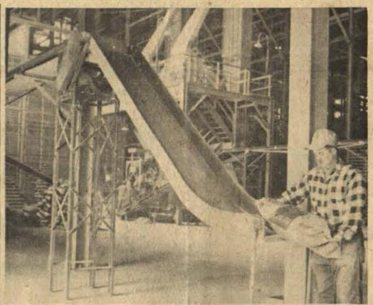
MANPOWER needed here. This is the end of the conveyor belt for sacked fertilizer. The man receives the sacks and stacks them on a wooden platform or pallet. The load is shifted to storage or to the shipping floor by fork lift trucks.
