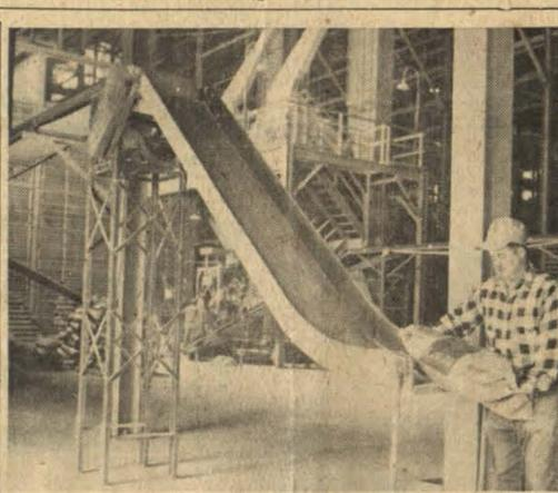
**MANPOWER** needed here. This is the end of the conveyor belt for sacked fertilizer. The man receives the sacks and stacks them on a wooden platform or pallet. The load is shifted to storage or to the shipping floor by fork lift trucks.
