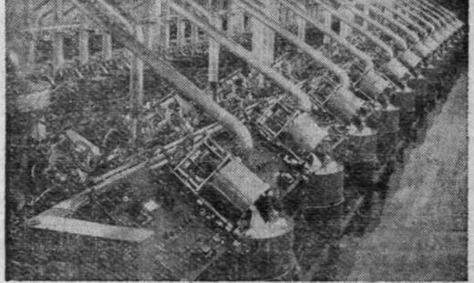
Part of the 226 electric eye sorting machines in operation at the bean terminals of the Michigan Elevator Exchange at Port Huron and Jackson.
