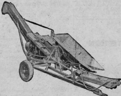
This outstanding machine can be compared with any on the market today. It has 70% larger husking capacity than the previous model, larger wagon elevator, more clearance on the ground, shells less corn because of improvements made in the snapping rolls. Picks tall corn, short corn, down corn or listed corn. After you see it you will agree it's the best in the field.
