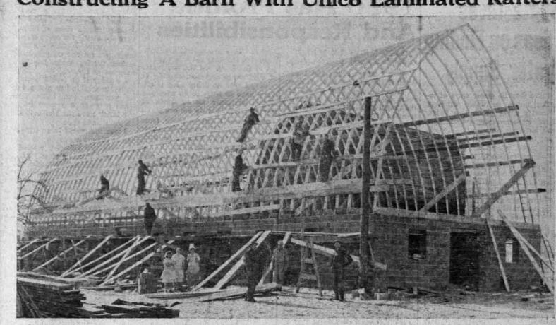
This is a typical scene that is going on throughout the state on many farms and from all indications will be intensified in the coming months ahead. This 30 f oot by 75 foot barn is being constructed with Farm Bureau Unico Laminated Wood Rafters on the John Schwab farm at Bay City. The rafters are engineered for immediate erection and provide low cost construction. Mr. Schwab is shown standing on the left of the two workmen in the foreground.
