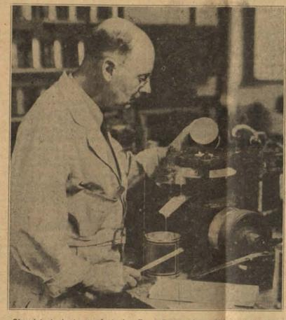
Chemist at glant manufacturing Farm Bureau Soya Paints demonstrating the grinding process in the manufacture of paints containing soya oil from American grown soy beans. The miniature stone mill shown above is an exact model of the large mills used in the factory to grind paint ingredients, pigments and oil together in a smooth, fine and permanent union.
