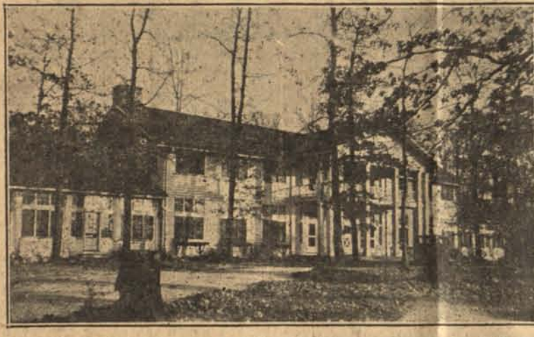
Cromaine Hall is the center of the Waldenwoods group of buildings. It houses the assembly room, dining hall and men's dormitory.
