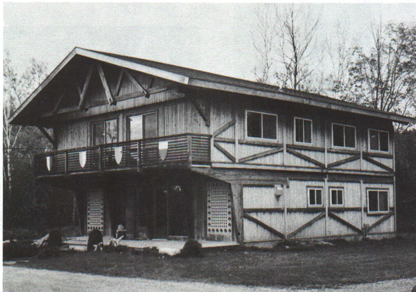
Small office building built largely of cedar. Cedar's decay resistance gives it an advantage over most other woods for exterior applications such as these.
