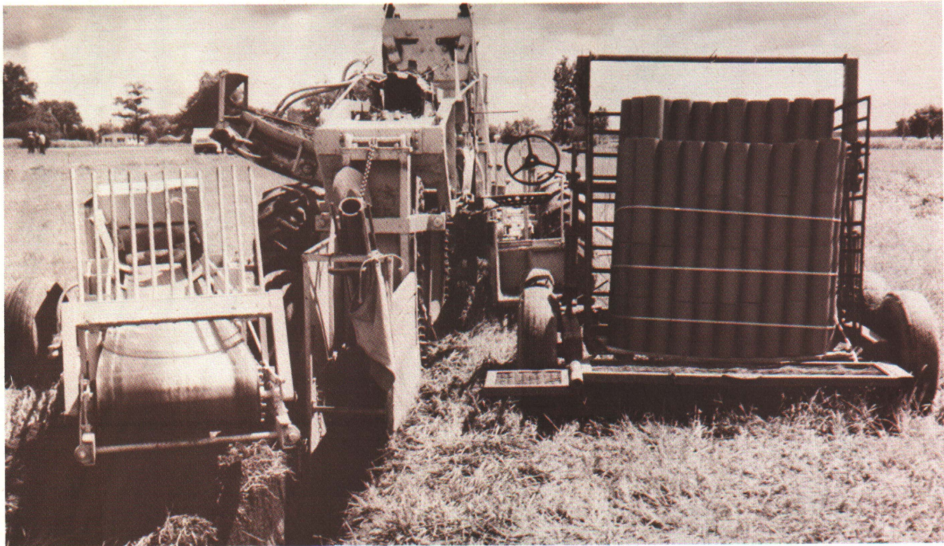
Thousands of acres of crop land in Michigan would produce higher yields if the soil were better drained. This wheel type trencher was used to install tile on the Saginaw Valley Bean and Beet Research Farm.
