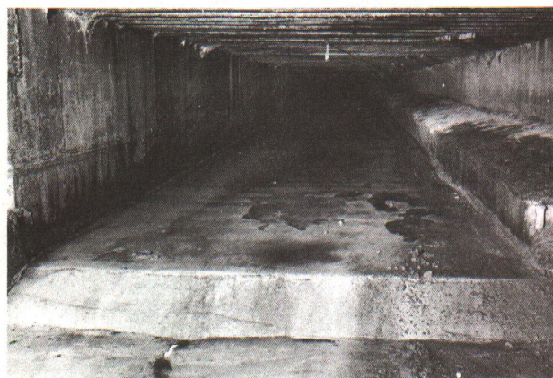
Fig. 9. Before (left) and after (right) flushing. The raised surface (right in both photos) is directly under the center alley of a completely slotted floor. A row of concrete blocks laid the length of the trench and capped to form a sloped surface permits the alley to be hosed off as needed. By narrowing the trench, the flush water is confined to the manure area and less water is required.
