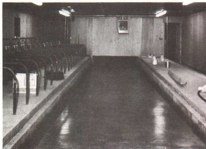
Fig. 4. A concrete sealer helps prevent manure from adhering to the surface of the trench. Make sure the building is well ventilated when applying a polyurethane product.
