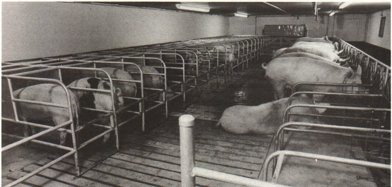
IN THE FLUSHING SYSTEM at the MSU Sow Gestation barn, floor. The front part of the stall is a solid strip of concrete. tank shown at the top of the photo.
