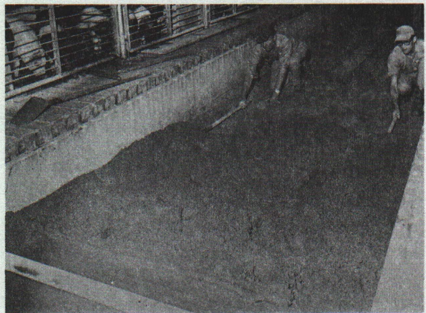
Fig. 7. Moving the pipes as pouring progresses. To maintain an even slope, make sure the pipes are always resting on 3 stakes.
