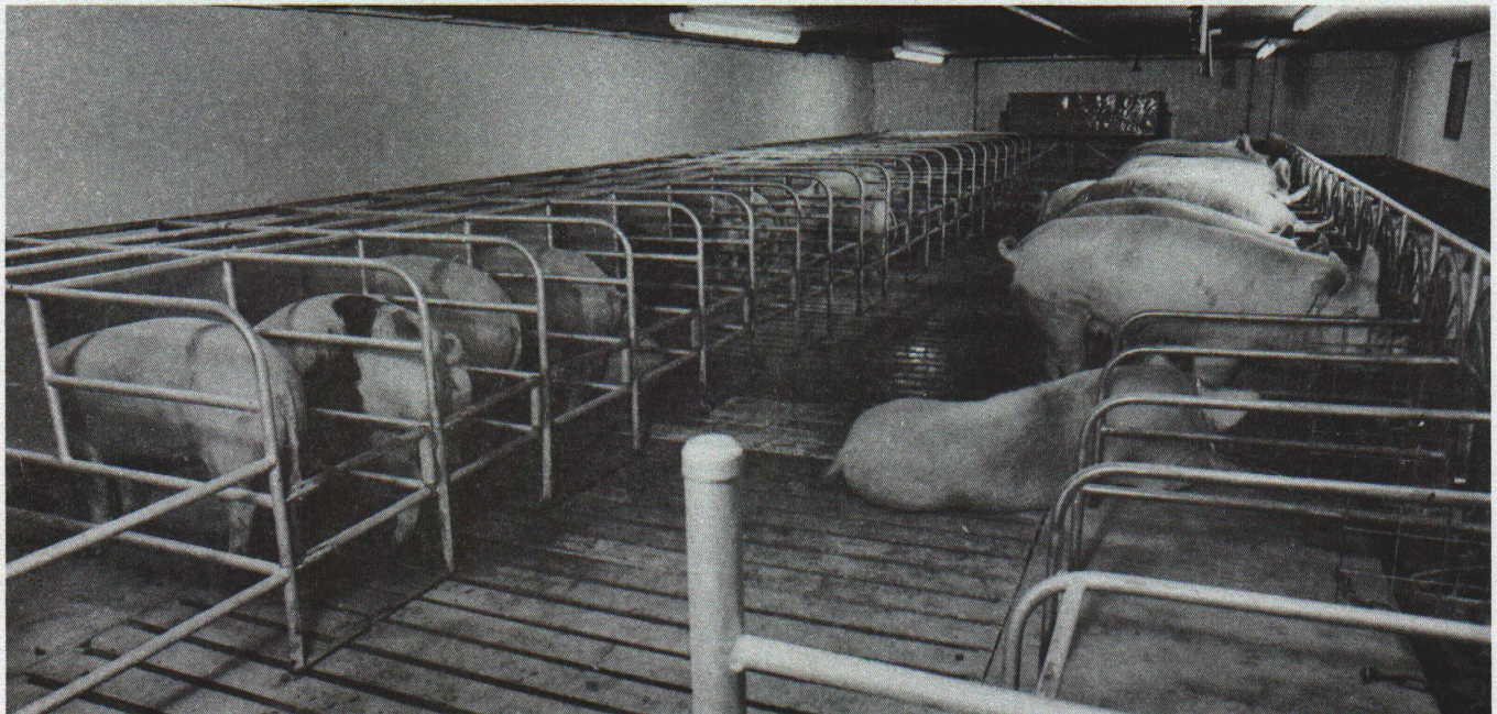
IN THE FLUSHING SYSTEM at the MSU Sow Gestation barn, the two rows of sows stand with their hind legs on an 8' slotted floor. The front part of the stall is a solid strip of concrete.
