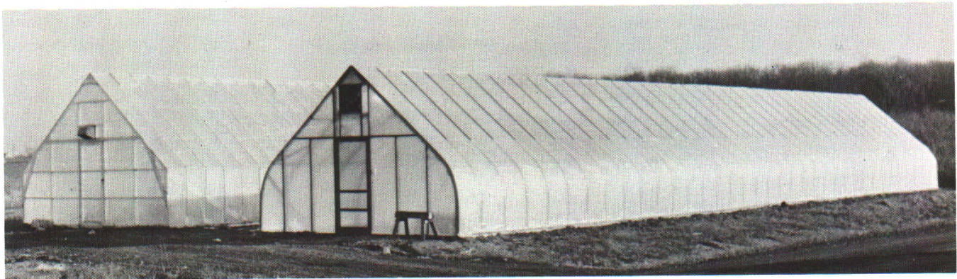
Flexible plastic film can be used for many types of greenhouse construction.
