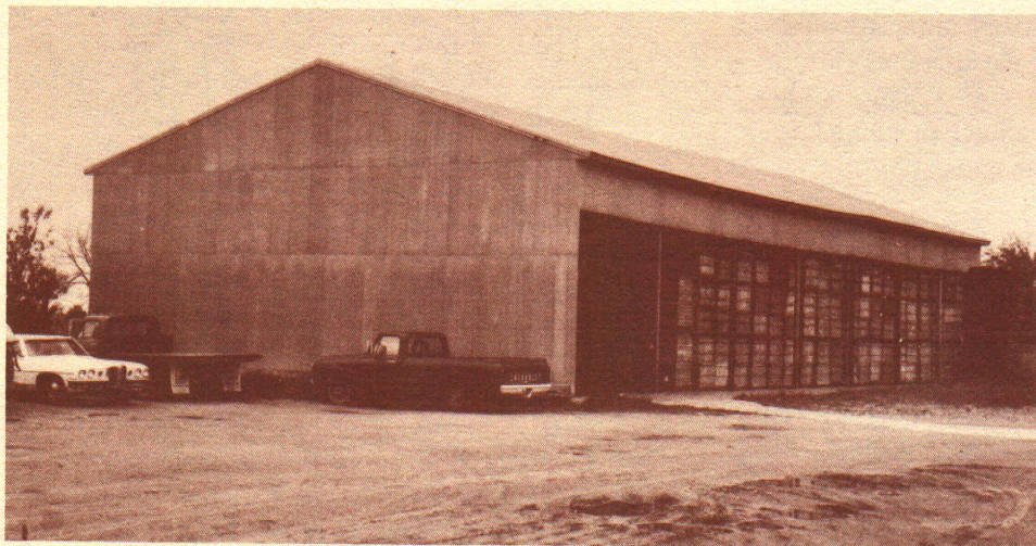
Pole type building for storage of boxes when they are not in use. This building protects the boxes and allows them to dry, reducing decay hazard.
