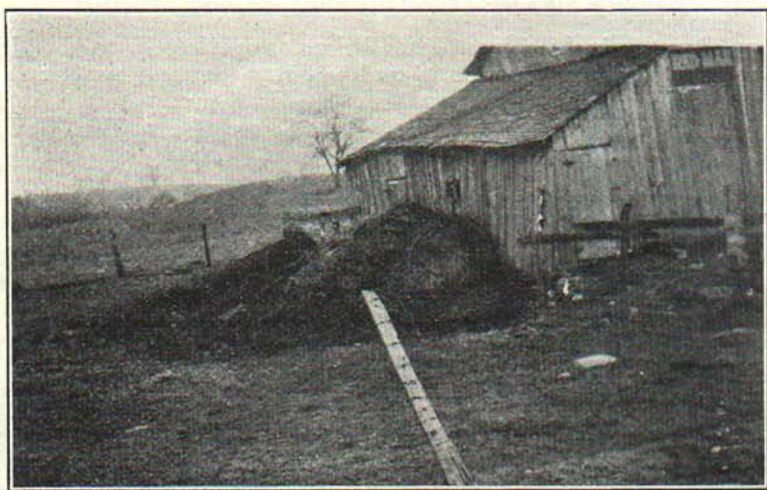
Fig. 5. Manure stored in this manner will suffer a large loss from leaching by water from the eaves.
