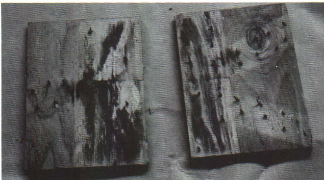
Figure 4 — Gusset plates taken from a truss showing the mold formed in the glue — indicates very little contact area.
