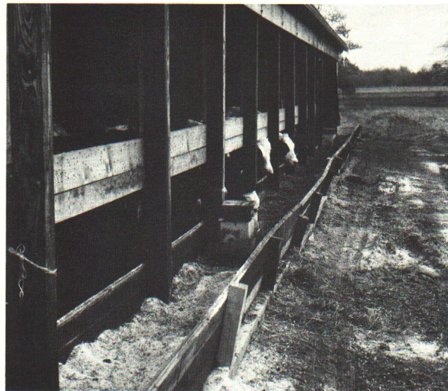
Figure 18 — Fenceline feeding bunk on the open side of a free stall youngstock building.
