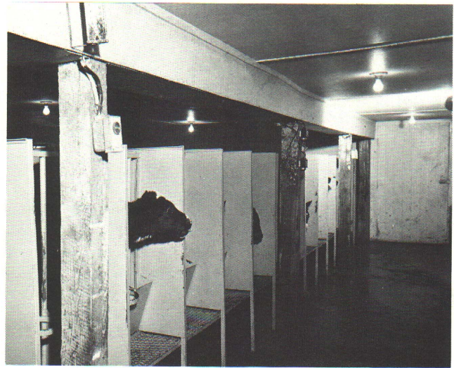
Figure 8—In warm housing, calves can be raised on slats. Water is used to clean so facilities for handling liquid manure should be available.
