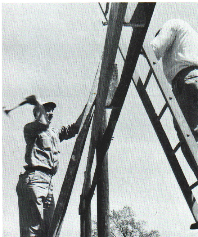
Vertical bridging is spiked secure between rafter supports at truss locations.
