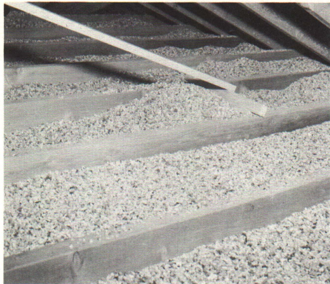
Figure 1. Leveling fill type insulation placed between ceiling joists.
