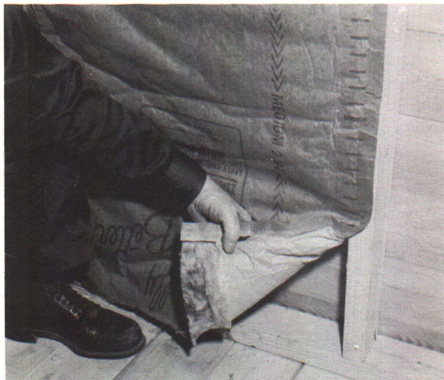
Figure 3. Providing a nailing flange at the bottom of blanket insulation for nailing to the sill.
