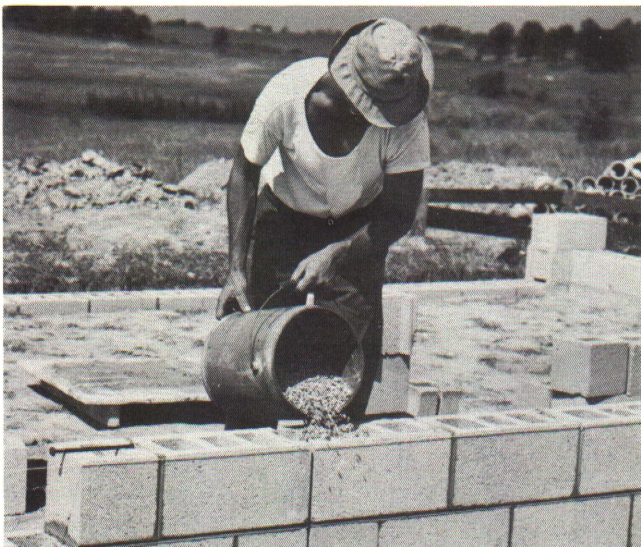
Figure 2. Pouring granular fill insulation into the cores of a block wall.
