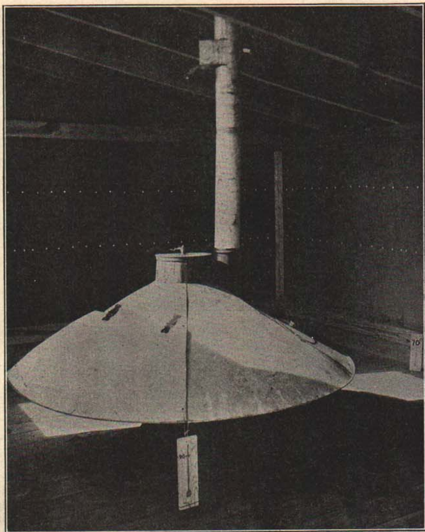
Fig. 3.—Proper location of thermometer. A temperature of 90° under edge of hover and a room temperature not to exceed 70° is ideal.
