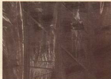
Fig. 19.—A plastic film vapor barrier is placed over all blanket insulation to provide double protection against vapor transfer into the wall materials.
