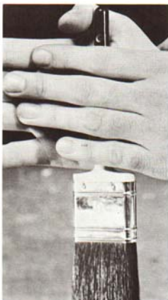
When cleaning a brush, remove most of the material in the appropriate solvent. Then twirl the brush, holding the handle as shown. This will remove most of the remaining solvent.
