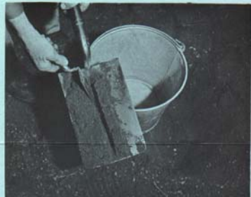
Using the trowel or similar tool to reduce the sample.
