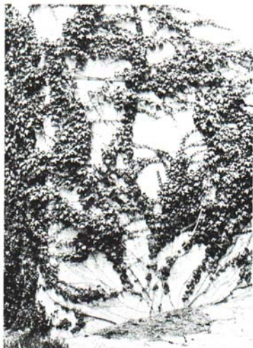
Fig. 13 Veitch Japanese Creeper climbing on masonry building.
