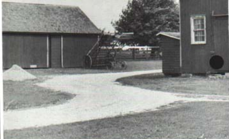
Fig. 21. Surfacing for the work-service area may be grass, gravel, crushed rock, or other durable material.
