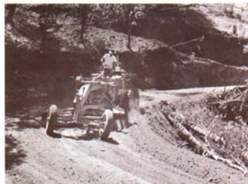
Fig. 4. Diesel motor grader (50 brake horsepower) working on logging road. This machine, plus one 75-horsepower diesel tractor, builds and maintains the access haul roads to the logging operation. (Photo: Caterpillar Tractor Co.)
