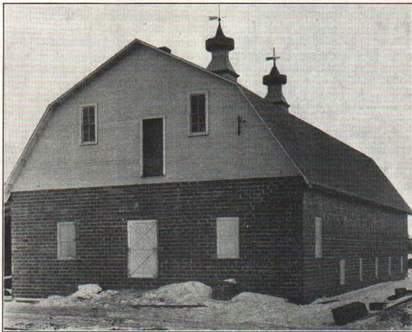
Fig. 4.—This 38 by 70 storage is similar in design to the one shown in Fig. 2. There are two eight-inch glazed tile walls with a two-inch air space between them. The height of the storage room is 14 feet, or about two feet higher than those shown in the other figures. The capacity is about 10,000 bushels. Note the large size ventilating cowls.
