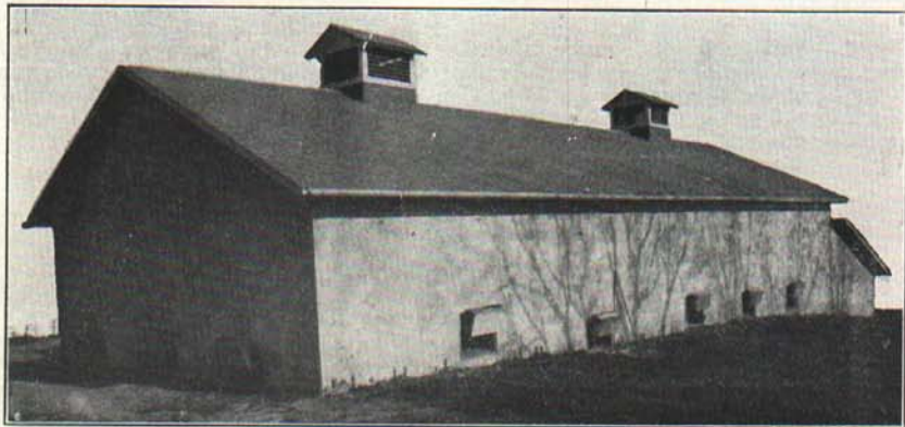
Fig. 3.—The walls of this storage consist of twelve inches of interlocking tile with waterproof plaster on both the inside and outside. It is 33 by 80 feet in size and has a capacity of 12,000 bushels. Hair felt is the principal insulating material of the ceiling. The air intakes are just above the ground line and are well distributed about the building. The air outlets are each 4 by 4½ feet.
