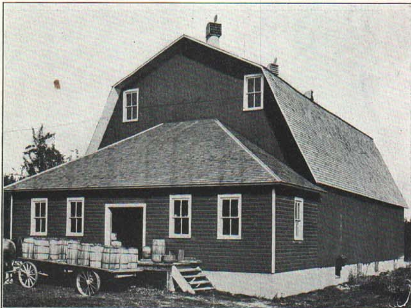
Fig. 1.—This frame storage was built in 1922. It is 40 by 60 feet and has a capacity of 10,000 bushels. A grading room extends across the front. The second floor is used as a storage for empty containers. This is one of the few storages in Michigan with a permanent false floor. A two-inch thickness of hair felt in the walls provides excellent insulation. Note the location of air intakes and outlets.
