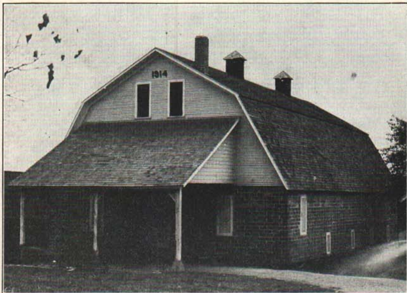
Fig. 2.—One of the older air-cooled storages of the modern type. The size is 36 by 60 feet, including a nine-foot sorting room across the front, and the capacity is about 8,000 bushels. There is an outer wall of eight-inch glazed tile and an inner one four inches thick and between the two is an insulating quilt. The second floor is used for the storage of empty containers.
