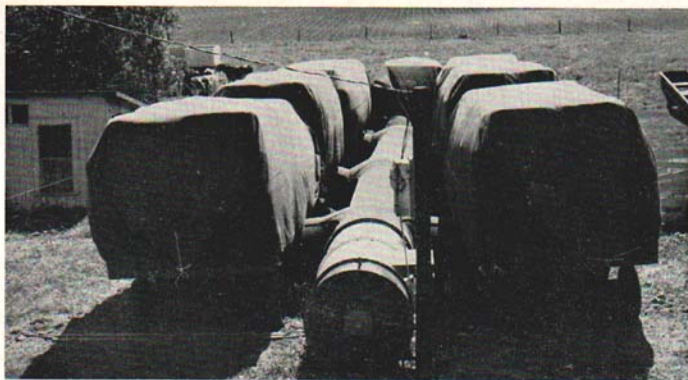
FIG. 16.—Wagon drying baled hay.
