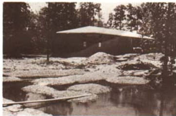
Fig. 8 — Septic tank disposal fields will fail and basements may be wet on soils with mottled or gray subsoil and slow permeability.
