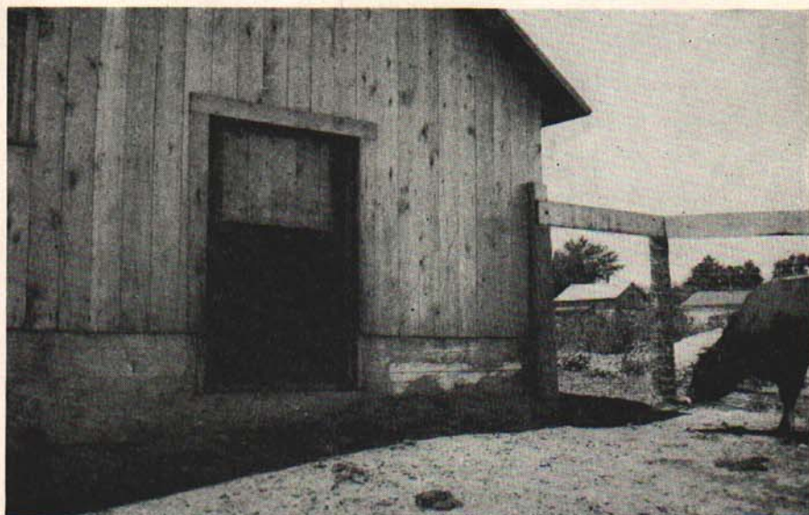
Fig. 9. A vertical-sliding door is not easily damaged by the bull.
