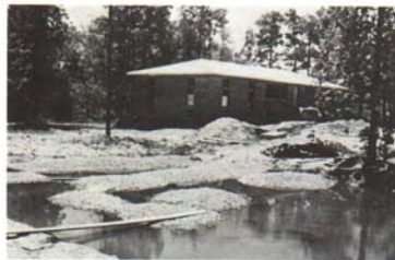
Fig. 8 — Septic tank disposal fields will fail and basements may be wet on soils with mottled or gray subsoil and slow permeability.
