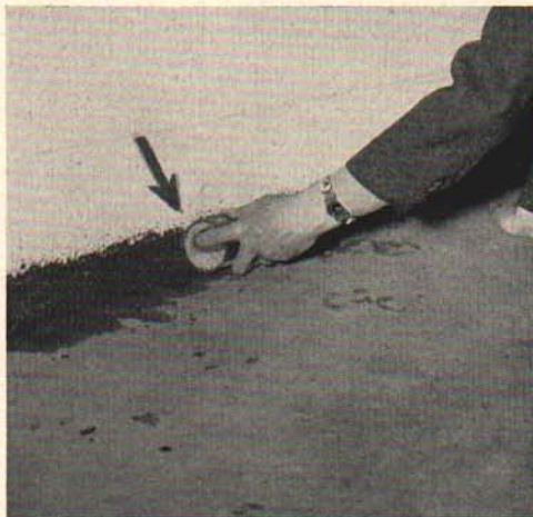
Fig. 7. A cove can be made between the wall and floor with an ordinary milk bottle as a tool.
