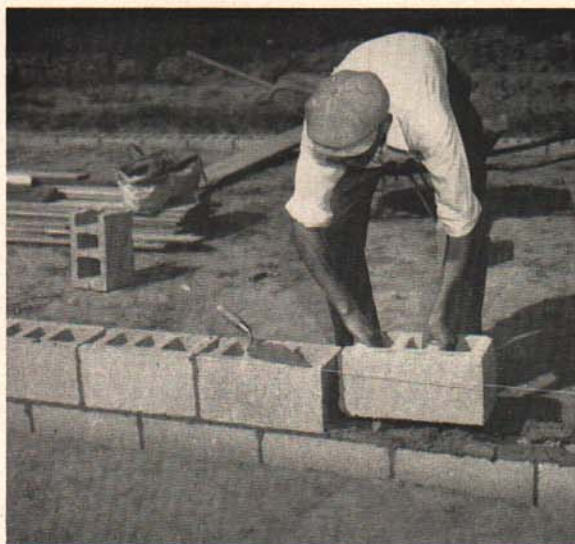
Fig. 18. Using a chalk line to line up the rows of blocks between the corners.
