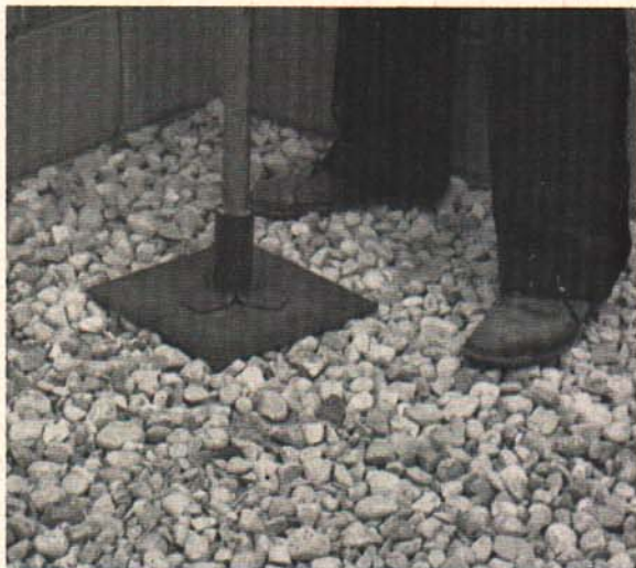
Fig. 10. Compacting the gravel fill for a dry, warm floor.
