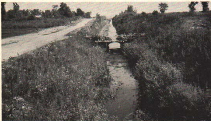
Fig. 3. The master dam in the main Chandlers Marsh drain, 3 miles north of East Lansing. It is constructed of a 7-foot tube of corrugated sheet iron 28 feet long, with tube filled over with soil to form a bridge. Some clay is necessary in the fill to prevent seepage and possible undermining. The dam is open in the early fall (photographed September 26, 1950) to lower the water level, and give more drainage for the extensive sugar beet acreage on the muck above. Note the weed growth below the dam (foreground), and the weed-free channel above.
