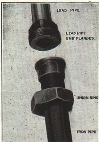
Figure 9: Lead pipe can be attached to iron pipe by an ordinary union.
