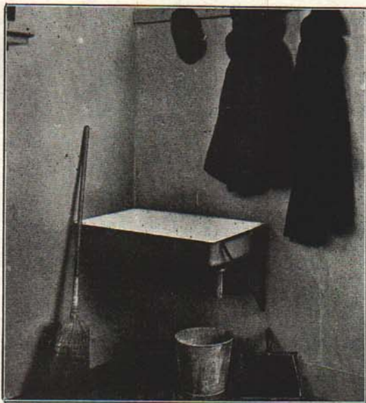
Figure 1: A sink improperly located with an inadequate method of sewage disposal. It is of little value.
