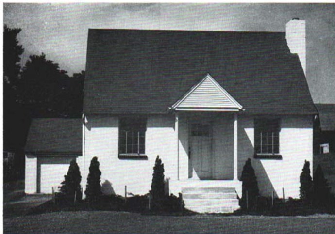
Fig. 6. Concrete blocks can be used to good advantage in the construction of farm houses.
