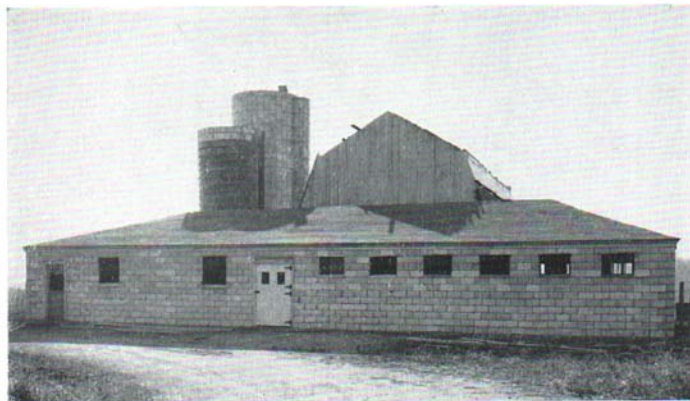
Fig. 7. Single-story dairy barns of concrete block construction are fire-resistant and serviceable.
