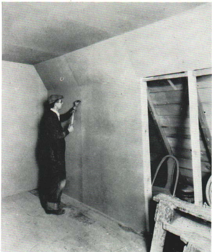
Fig. 6. Four-foot sheets of rigid insulation applied to inside surface of wall studs and ceiling rafters.
