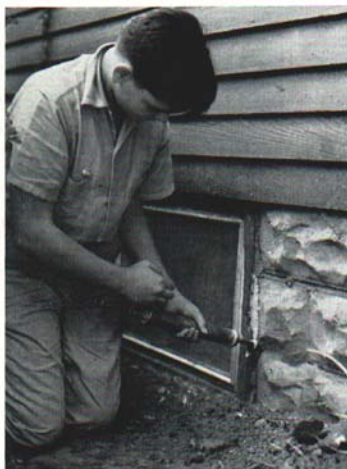
Fig. 3. Using a caulking gun to fill cracks between window frame and masonry wall with caulking compound.
