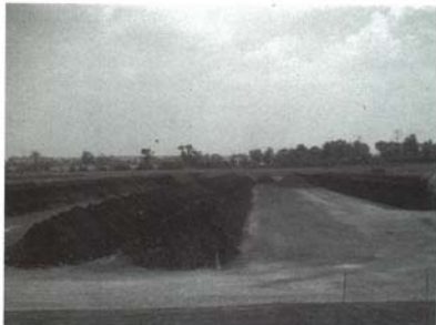
A firm pad base makes a weatherproof composting area
