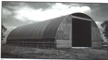
Figure 1 Typical hoop structure.
