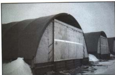
Figure 5. Closed end of hoop during cold weather.
