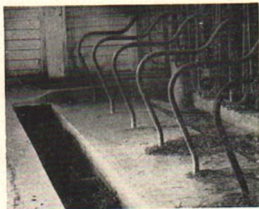
Fig. 23. (Above) Corner over-pass. Before the operator starts the cleaner, all manure is scraped into the gutter.
