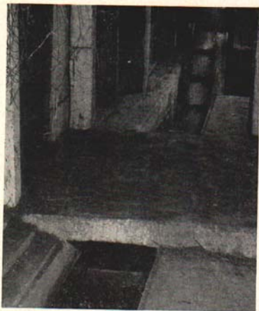
Fig. 21. Over-pass at the end. Note grooves on the top of the gutter for cover plates. Elevator and drive shaft in background.
