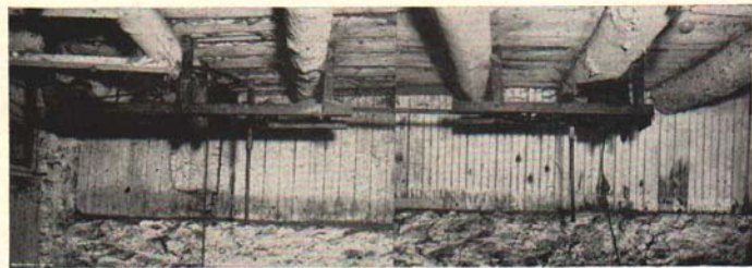
Fig. 8. The interior view of a dairy barn, showing the apron-return arrangement using one motor to operate two drums. Clutches are friction-disk type.
