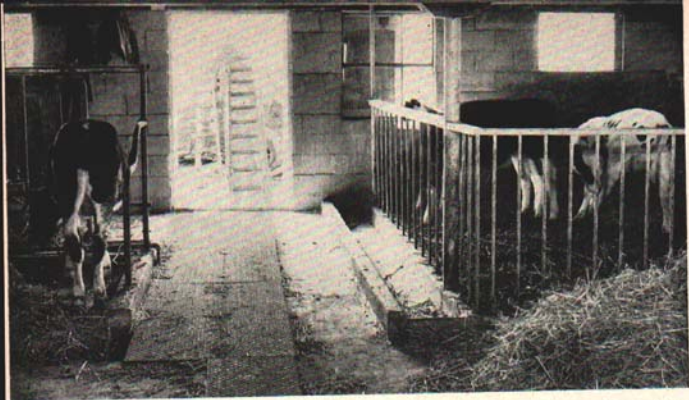
Fig. 22. (Above) Metal over-pass for cleaner across drive. Elevator in background. Farrell farm near Williamston.
