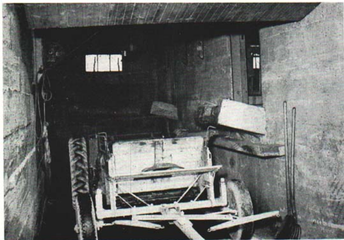
Fig. 9. The spreader is housed in a ramp at one end of the barn ready for use. The ends of the gutters extend out from the wall on the right-hand side.
