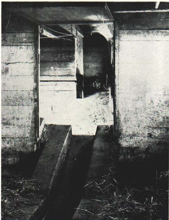
Fig. 8. A slight incline at the end of the gutter raises the manure high enough to drop directly into the spreader on the Hansen farm.
