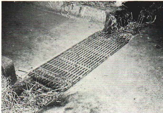
Fig. 5. A grate used over the gutter at a crosswalk to permit the gutter and conveyor to continue straight through the barn.
