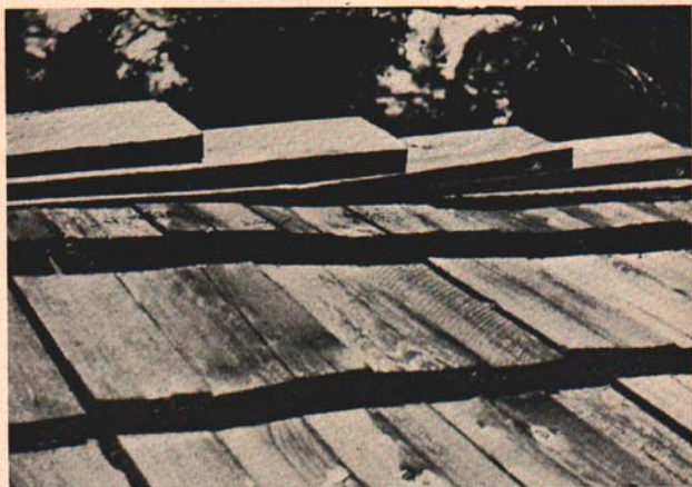
Fig. 17. Detail of lapped shingle ridge roll.
