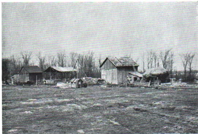
Fig. 1. These buildings are being replaced by new ones constructed of native material.
