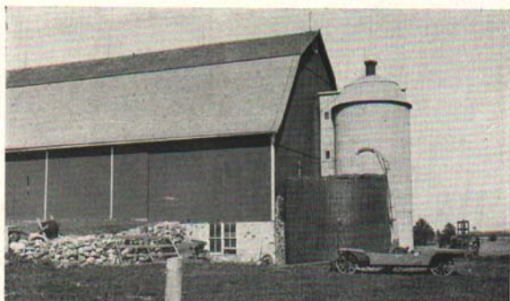
(Courtesy of American Lumberman.) Fig. 2. A temporary crib silo beside a permanent silo.
