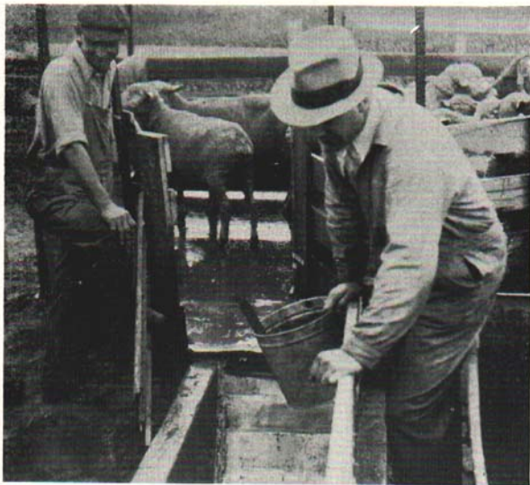
Fig. 16. A permanent concrete dipping tank. Many of these tanks are constructed on a community basis and large numbers of sheep are dipped cooperatively.
