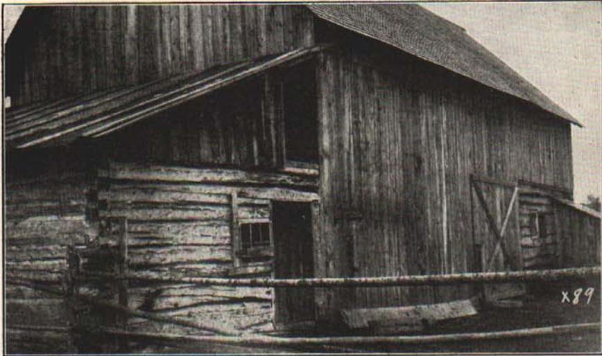
Fig. 7.—A barn near Republic. The logs and lumber all came from the farm, the lumber being sawed at a local mill. The horse and cow barns are in opposite ends of the building, making unhandy care and feeding. There are also too few windows.
