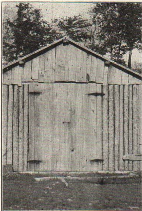
Fig. 11.—A garage made of tamarack poles. This method shows larger chinks, which are harder to fill than those in buildings where the poles are trimmed on each side.
