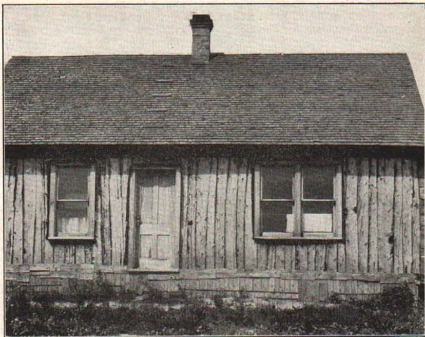
Fig. 8.—A house made of cedar logs, hewn and set on end.
