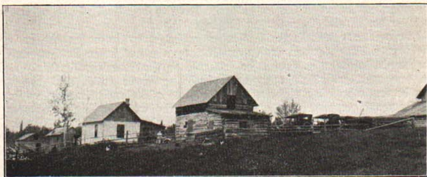
Fig. 4.—A complete set of farm buildings near Republic, Michigan, built of logs and lumber sawed on the farm. The cost of these buildings, not counting the owner's labor, was about $450. A better arrangement of the buildings would have added to the convenience of the farm and made possible better use of the log houses when permanent buildings were erected.
