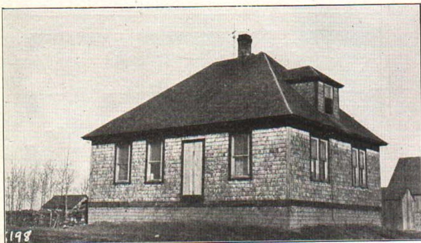
Fig. 14.—This house was made of cedar logs, as was the house in Fig. 8. The logs were then covered with shingles, making a neat and weatherproof home.
