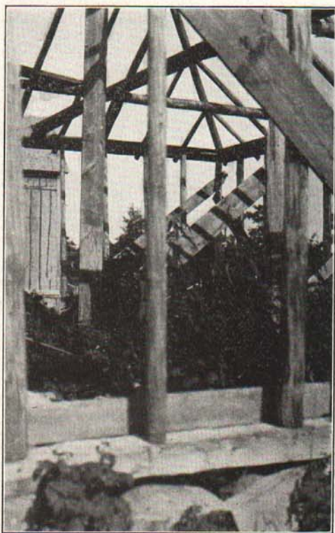
Fig. 6.—A corner of framework made from spruce and tamarack poles. The poles are toenailed to the hewn log used for a sill.
