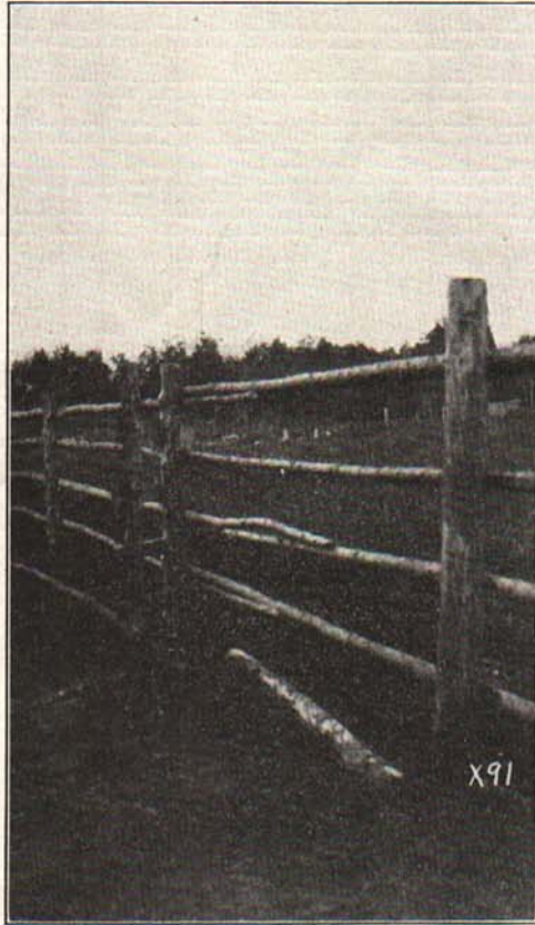
Fig. 30.—Poles make a serviceable temporary fence.
