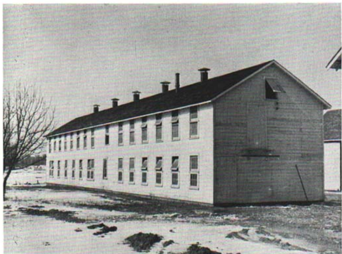
Fig. 8. This house was a one-story shed-roof type laying house. When the roof had to be replaced, the owner, needing more laying house space, built a second story. The top story has a straw loft, the lower story is ventilated with windows. The entire house is well-insulated.
