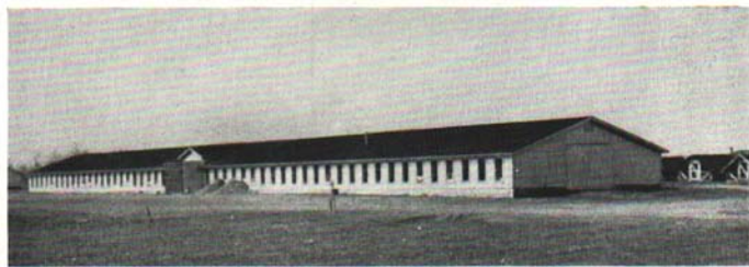
Fig. 4. A 30' x 210' laying house which has a 10-foot feed room in the center making a pen on each side 30' x 100' feet. This laying house houses 3,000 Leghorns, is well-insulated with heavy insulation board and is covered with a built-up roof.
