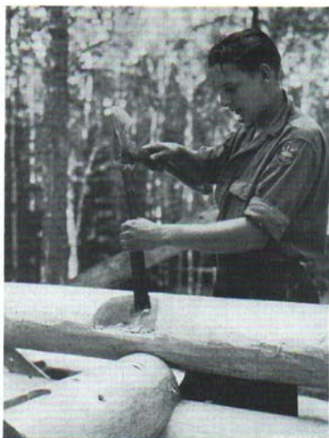
Fig. 8b. Notching logs with a heavy gouge. (Photograph by U. S. Forest Service.)
