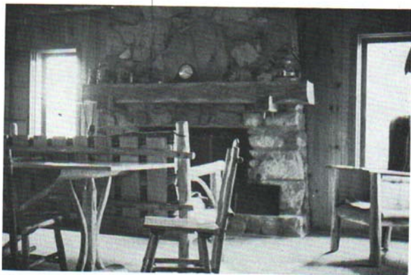
Fig. 20. Interior finished in knotty pine lumber. Note the odd character of the furniture, the massive hewed mantelpiece, and the level of the hearth.
