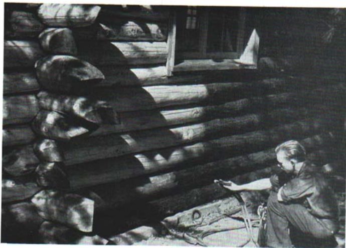
Fig. 25. Treating the exterior with a creosote stain.
