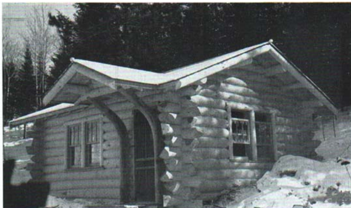
Fig. 15. A well-appointed small log cottage. Note the width of the eaves and the unusual method of supporting the porch roof. (Photograph by U. S. Forest Service.)
