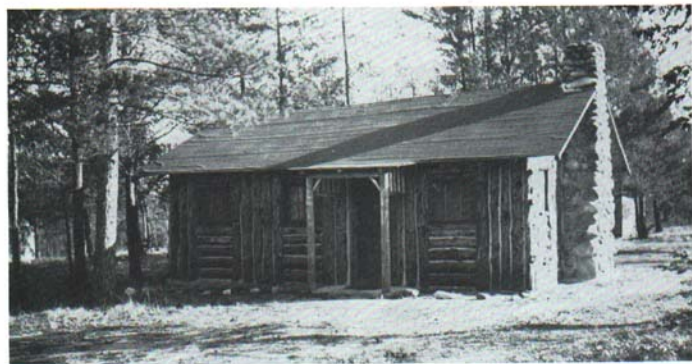
Fig. 10. An attractive combination of vertical and horizontal logs. Extreme knottiness produces a very unusual effect. The general appearance would be vastly improved by shingling the roof.
