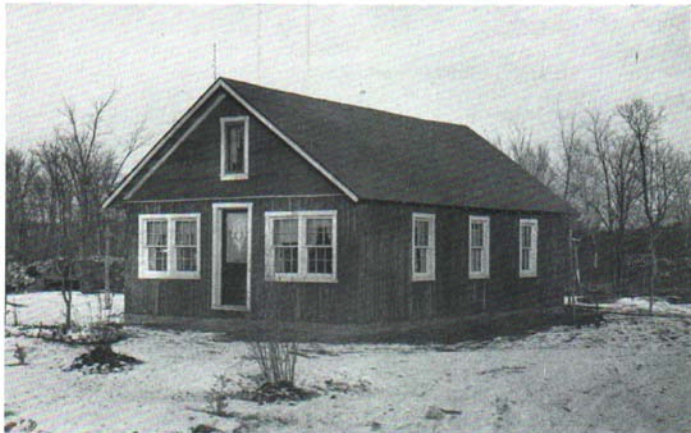
Fig. 11. A "split-log" cabin of modest design. The building would be much more attractive with a shingled roof and gabled end, a more suitable door, a porch, and a bit of shrubbery around the foundation. (Photograph by University of Wisconsin.)
