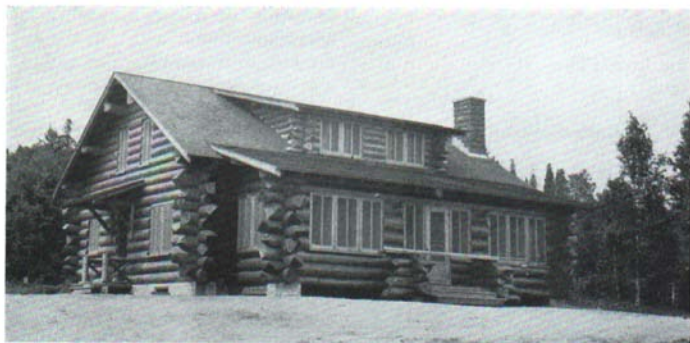
Fig. 3. A well constructed horizontal log house of Norway pine. The appearance might have been improved by facing the foundation and chimney with native rock. (Photograph by the U. S. Forest Service.)
