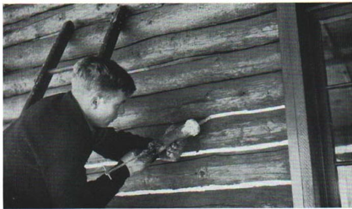
Fig. 26. Applying caulking compound with a pressure gun.
