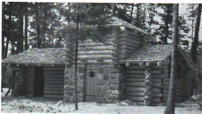
Fig. 21. Logs and rocks blend together in any type of building. Both were obtained locally as were the cedar shakes in the roof.
