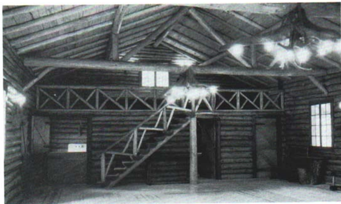
Fig. 24. Interior of a community cabin. Over any wide spans roof timbers must be braced. Note the rustic staircase, lighting fixtures and furniture.
